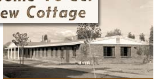
Marshall Cottage was designed by Place & Place Architects and named after the Marshall Foundation which contributed $50,000 towards the construction of the new cottage
