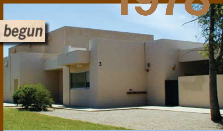
The Recreation Building was constructed, with a gymnasium, kitchen and arts & crafts rooms. In 2000, the Recreation building was dedicated in honor of Kent Richards.
